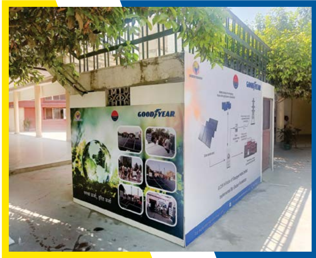
Battery room inside the Office of Commissioner of Police, Faridabad
